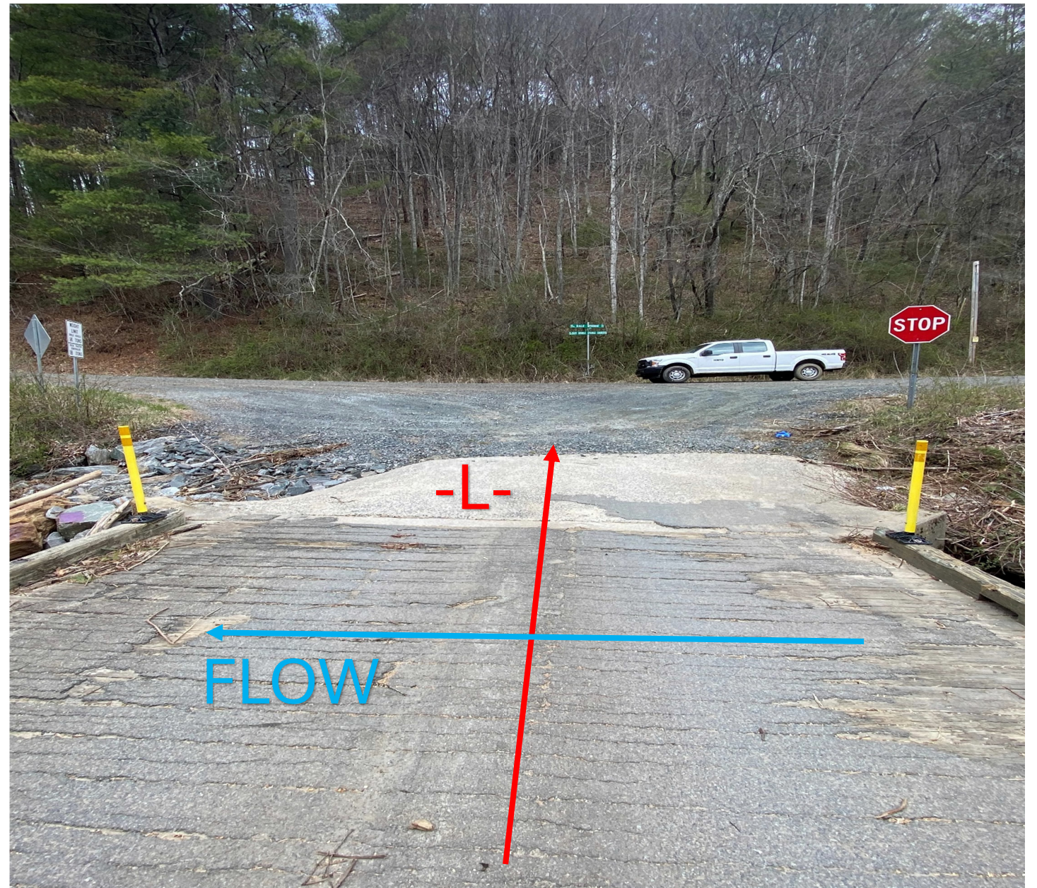
VIEW TO NORTHEAST FROM CENTER OF BRIDGE TOWARDS END BENT 2
